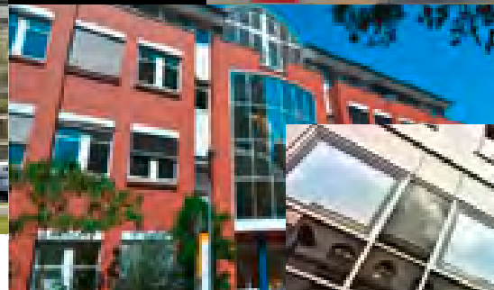
Office building with University of Bremen as main tenant
